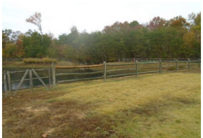
Fencing along McDaniel Road and around the water retention pond can have its life extended by replacing missing slats, straightening posts and screw fastening loose members.
